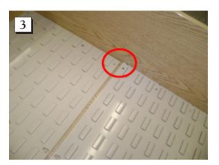
**Step 3.** Overlap the panels so that the two holes in the picture are on top of each other and repeat step 2.
