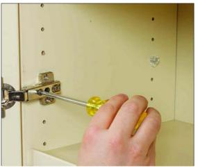
The left adjustment screw provides depth adjustment: Depth adjustment ... lets you bring any style of door into line with the vertical surface of the cabinet.
