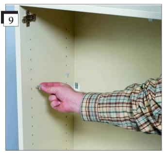
Decide the positioning of your shelf. The shelf is adjustable in  $1\frac{1}{2}$ " (32 mm) increments. Insert the clear plastic shelf pins in the back holes at your desired height. Once the back shelf pins are in place insert shelf pins into the front shelf holes at the same height as the back pins.
