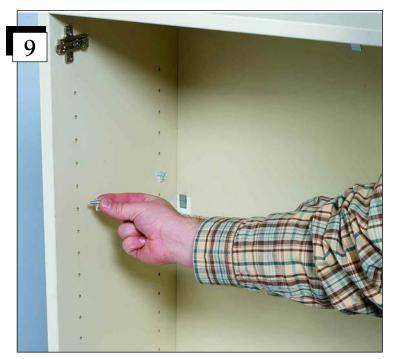
Decide the positioning of your shelf. The shelf is adjustable in 14" (32 mm) increments. Insert the clear plastic shelf pins in the back holes at your desired height. Once the back shelf pins are in place insert shelf pins into the front shelf holes at the same height as the back pins.
