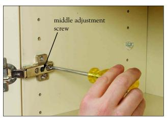
The right adjustment screw provides side adjustment: Side adjustment ... regulates the gaps between doors, cabinets and walls for perfect parallel alignment.
