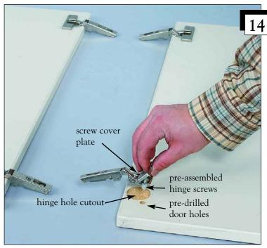
Begin by laying the doors flat on the ground with the hinge hole cutouts (inside of doors) facing up. With screw cover plate lifted, insert pre-assembled hinge screws into the pre-drilled door holes. There are two latches per door.
