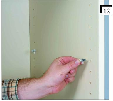
Once the back shelf pins are in place insert shelf pins into the front shelf holes at the same height as the back pins. Repeat steps for the opposite side keeping pins at the same height.
