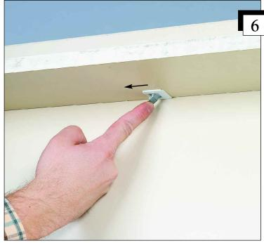
Once the toe and bottom panels are together, press the fitting toggles down to secure.
