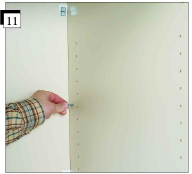
Decide the positioning of your shelves. Each shelf is adjustable in  $1\frac{1}{3}$ " (32 mm) increments. Insert the clear plastic shelf pins in the back holes at your desired height.
