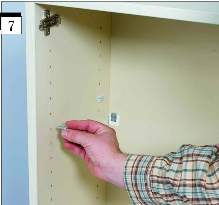
Stand your unit to the upright position. Decide the positioning of your shelf. The shelf is adjustable in 1/4" (32 mm) increments. Insert the clear plastic shelf pins in the back holes at your desired height. Once the back shelf pins are in place insert shelf pins into the front shelf holes at the same height as the back pins.
