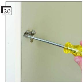
Position the latch over the drilled holes so the hook is on top. Using a Phillips screwdriver, insert the screws provided into the latch holes. Your latch is now secured to the door.
