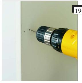
Drill the holes using a 1/8" drill bit. You only need to drill a little bit into the door. CAUTION: Be careful not to drill all the way through the door. You may want to mark your drill bit with tape as a guide so you do not drill too far.
