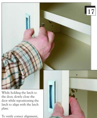
squeeze the latch lever to slide the hook under the latch. The latch should be able to catch.
