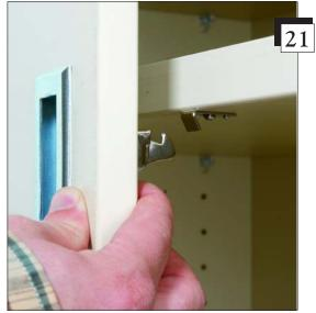
Your doors are now attached and ready for use. To close the left door, squeeze the latch lever and slide the hook under the latch plate. The latch will catch and secure the door.
