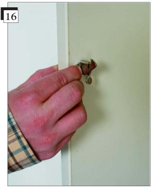
The door latch will attach to the left door. Hold the latch against the door with the hook at the top. Position it at a height even with the latch plate mounted on the shelf.
