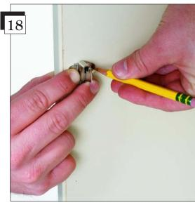
Be careful not to move the latch and open the door. Mark the mounting holes in the latch with a pencil. These markings will identify where to drill the holes to attach the latch.
