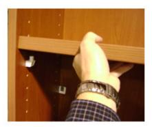
**Step 19.** Position the shelf on the clear back shelf pins. Make sure the white front shelf blacks line up with the holes in the shelf and LIGHTLY tap on the front of the shelf to slide onto blocks.
