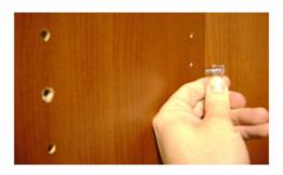
**Step 17.** Decide the positioning of your shelves. Each shelf is adjustable in 1½" increments and can be tilted up or down by using a different level of holes in the back. Insert the clear plastic shelf pin in the back hole at your desired height.
