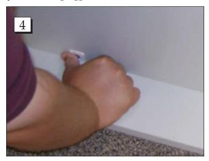
**Step 4.** Once together, press the fitting toggles down to secure.
