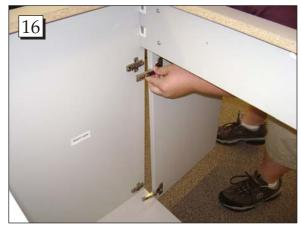
**Step 16.** Doors are ready to be attached. Position the left door onto the side of the cabinet unit. The hinges should align with pre-installed hinge plates mounted inside of the unit.
