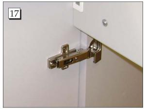
**Step 17.** Attach the hinges to the hinge plates by guiding the hooked area of the hinges around the small posts on the hinge plates and pressing them to the plates until they latch.
