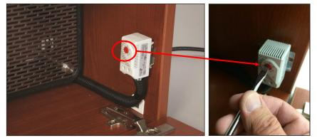
**Step 1.** Use a straight head screwdriver to preset cabinet to the desired temperature. Close the door and allow the unit to warm for 24 hours.
