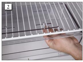
**Step 2.** Thread screw from the inside of the box through the rack into the retention plate - (trap refrigerator rack between box and retention plate).
