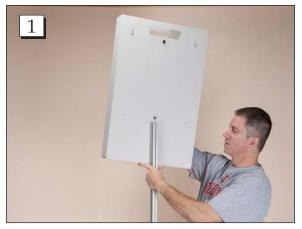
**Step 1.** Slide the T-Nuts on the protection organizer onto the pole.
