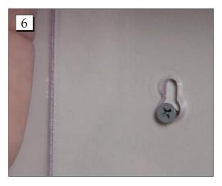
**Step 6.** Push the dispenser onto the screws through the largest part of the keyholes. Then pull the dispenser downward until the screws slide to the upper part of the keyhole.
