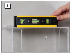
**Step 1.** Place the wall dispenser against the wall and use a level to straighten the dispenser.
