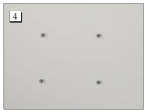
**Step 4.** Leave about  $\frac{1}{4}$ " of the screw out from the wall for the dispenser to hang from.
