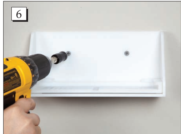
Step 6. Once level, tighten screws into the remaining holes.
