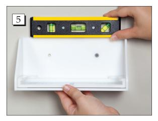
Step 5. Place a level on top of the Wall Mount.
